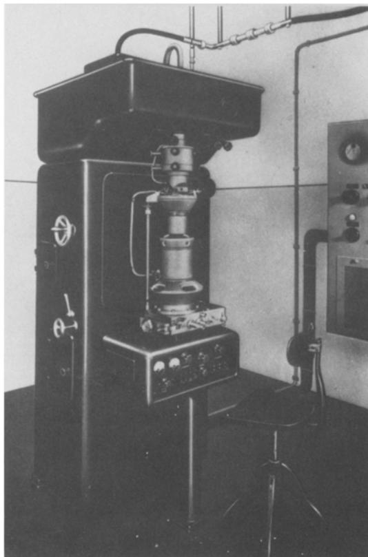
**Fig. 11.** The first serially produced electron microscope (Siemens). General view (21).
